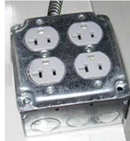
unregulated power junction box
