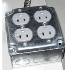
unregulated power junction box
